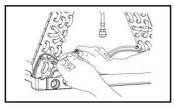
Figure 6. Removal of Orifice
